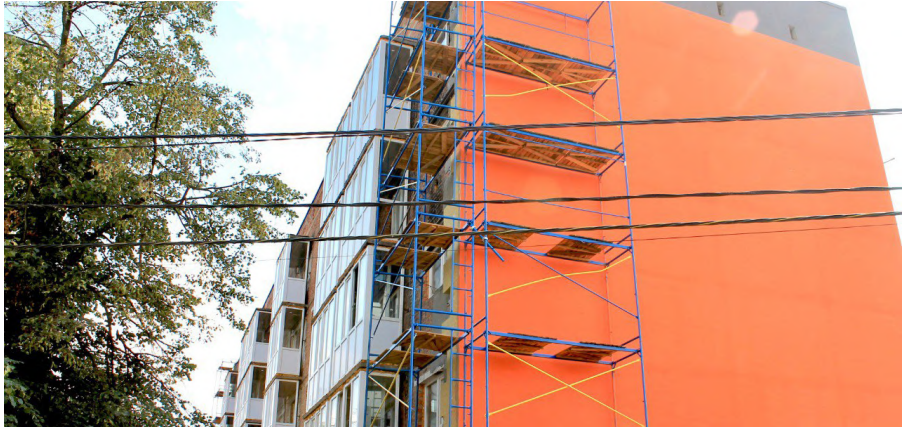
Restoration of a residential house in Trostianets, the Sumy region
